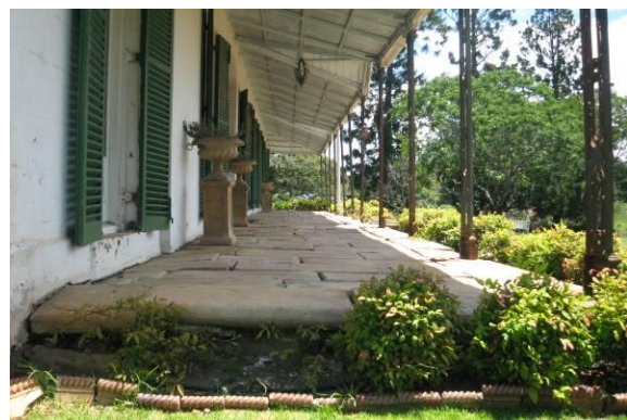
Figure 4.4 View of verandah to northern elevation showing uneven stone flagging.
