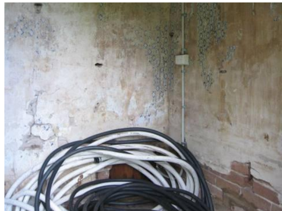
Figure 4.22 View of interior showing early wallpaper over the early plaster finish.
