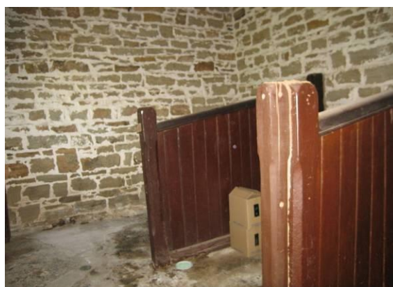
Figure 4.13 View of ground floor of stables—note the damp areas to the concrete floor and the boring activity in the front timber post.
