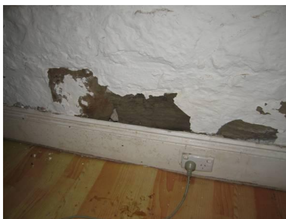
Figure 4.6 Damage caused by rising damp in the c1810 building.
