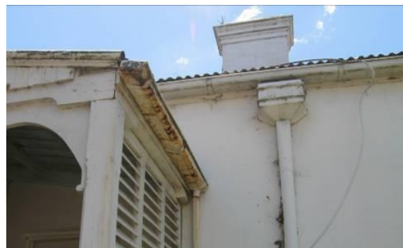
Figure 4.3 View of deterioration to gutters.
