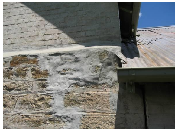
Figure 4.10 Section of eastern (rear) elevation showing inappropriate cement repair work.
